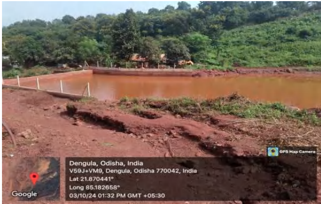
Figure 7.10: Check dam in foot hills of the existing Mine.
