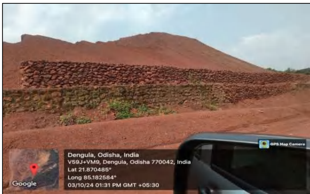
Figure 7.7: Retaining Walls along the Dump
