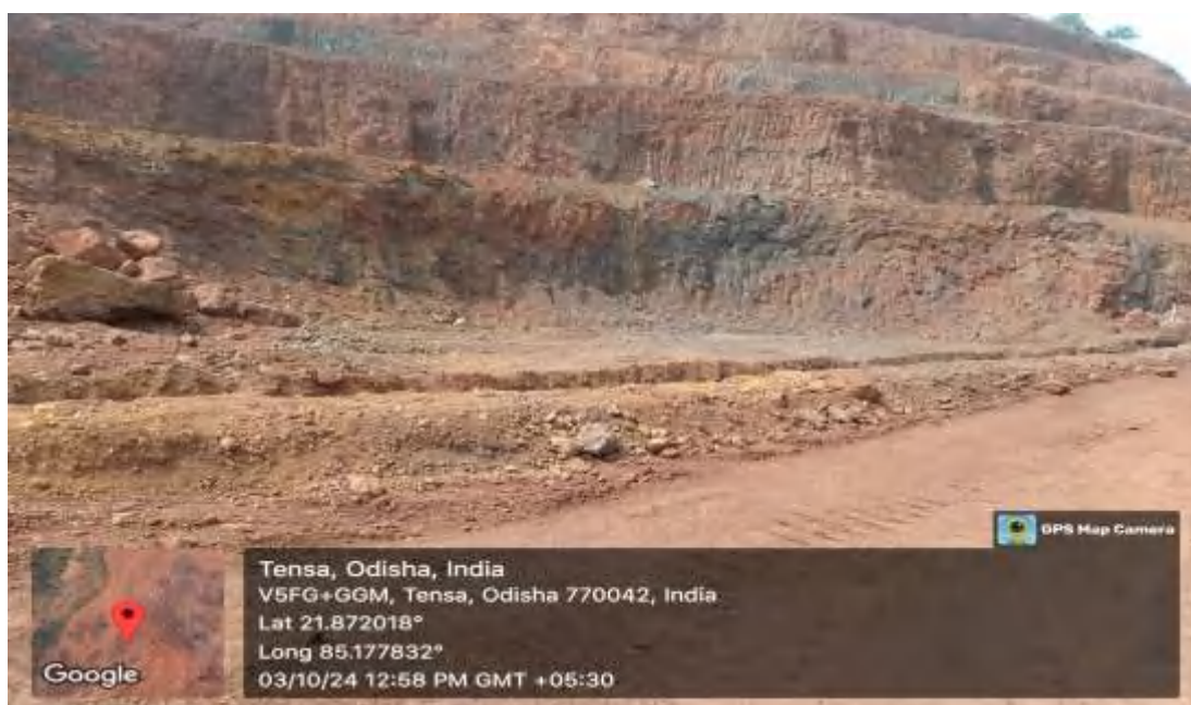
Figure 7.8: Garland drain from storm water in mining area.
