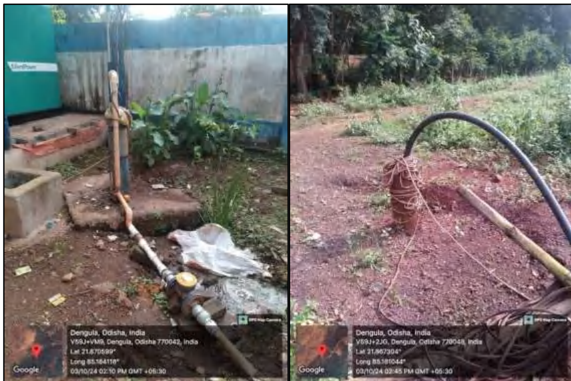
Figure 6.2: Groundwater withdrawal wells within lease area.
