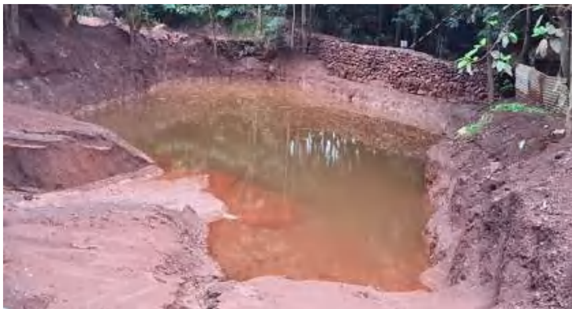
Fig-7.9: Rainwater Harvesting Pond
