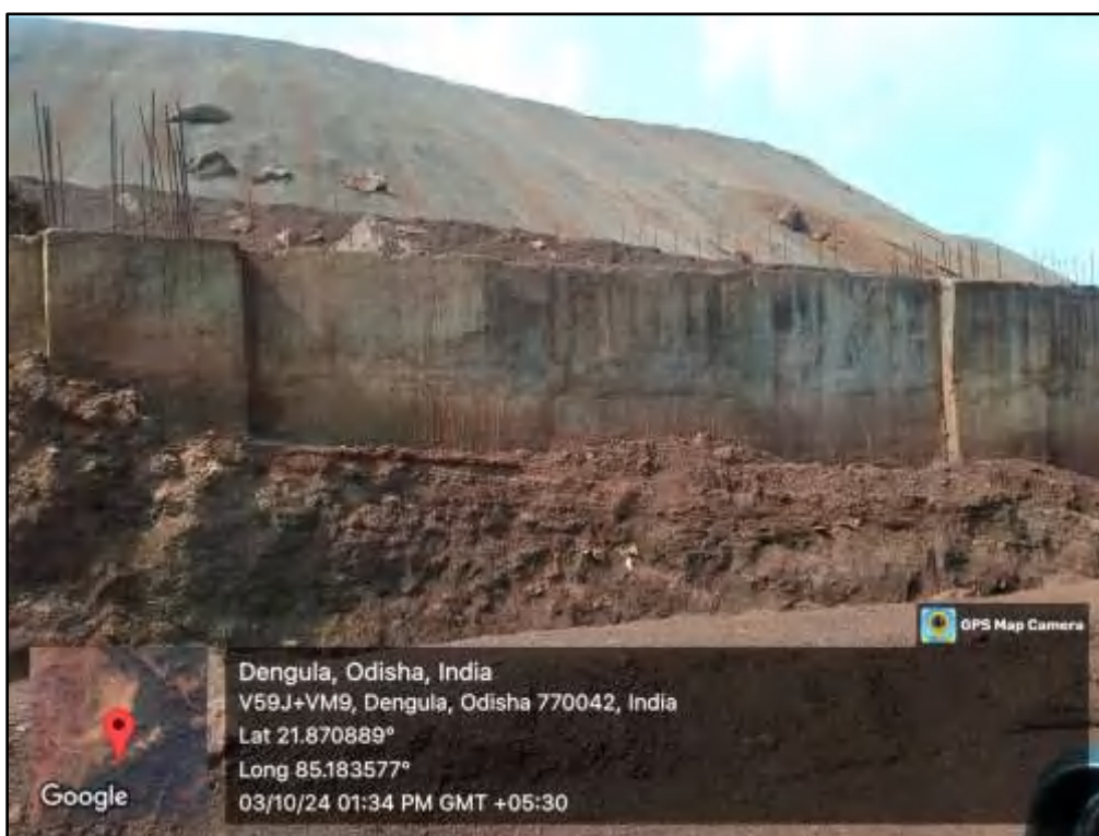
Figure 7.6: Concrete Retaining walls
